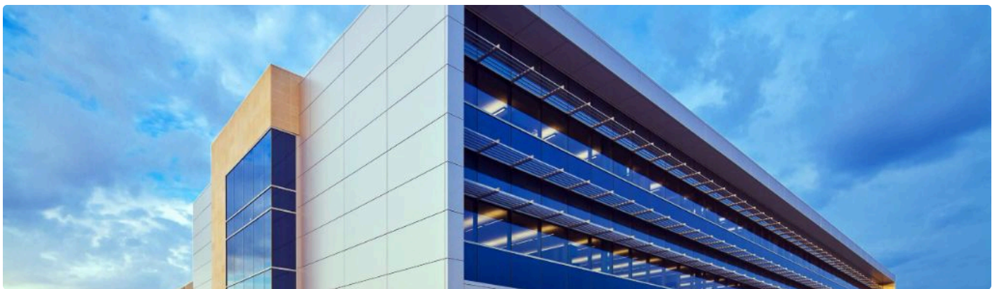
Modern commercial building infrastructure, the foundation for intelligent, connected, and vendor-agnostic Smart Building solutions powered by CorGrid®
